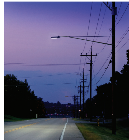
Retrofit existing utility poles
